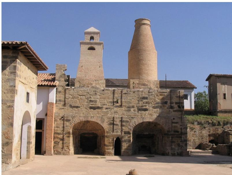
**Figure 1.** Twin blast furnaces, built in 1818, of the Iron Factory of São João de Ipanema. A vault was carved between the two furnaces in 1866. The upper part of the blast furnace on the right was altered in 1918. Image credited to Edgar Gomes (2006).
